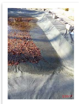
Use of cinder blocks is not a property way to secure a pool cover.
