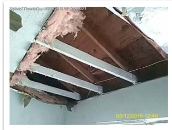
Treatment of studs with stain blocking primer.
