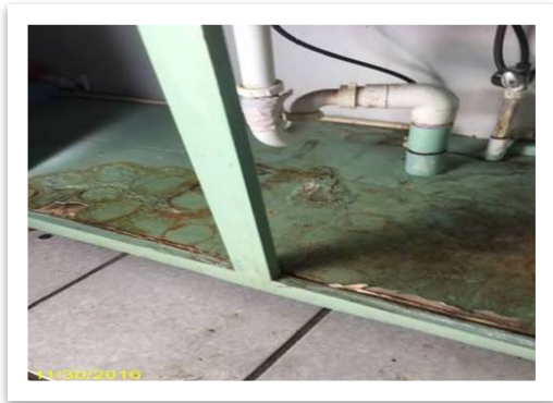
Chemical residue left under a sink.
