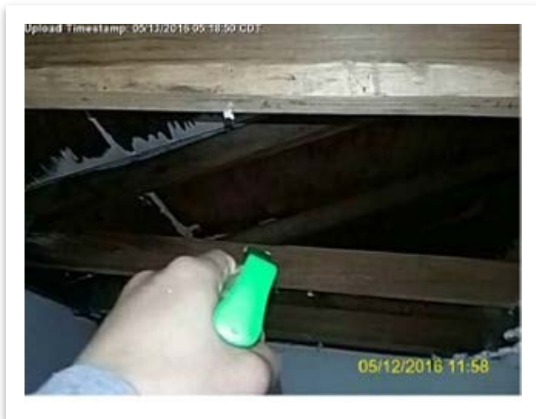
Treatment of studs with anti-microbial solution.
