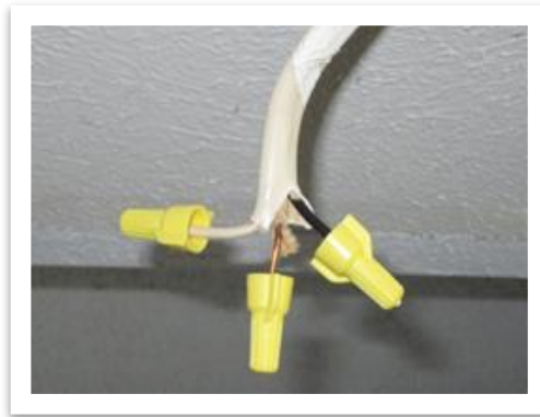
Example of Capping Wires
