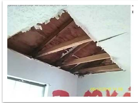
Removal of drywall and insulation.
